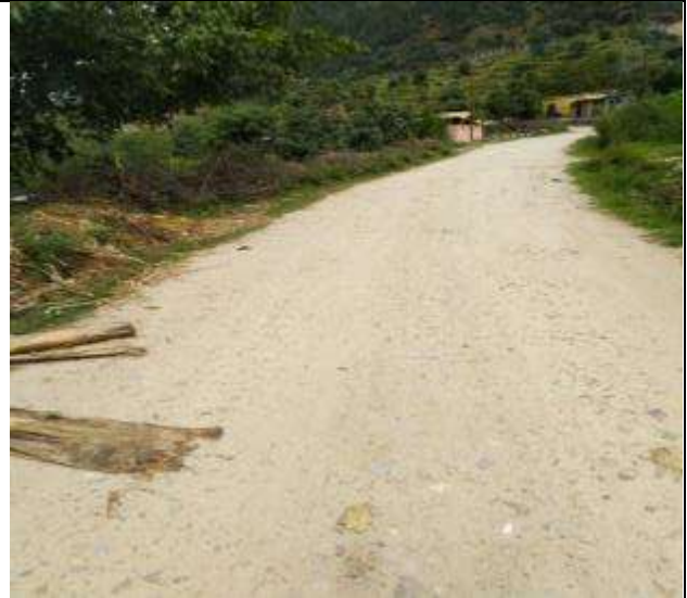
Condition of Road at Ch 0.0150 Km
