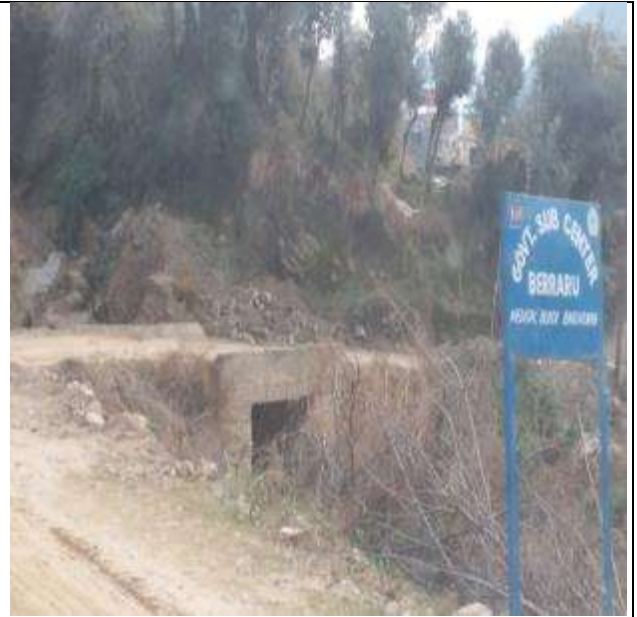
Sub Center at Berraru Ch 1.800 Km LHS
