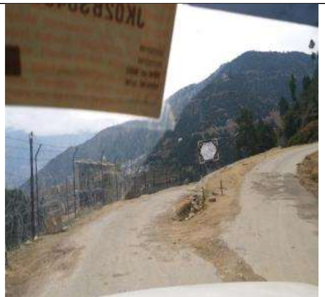
The project road diverts at Ch 3.900 Km RHS
