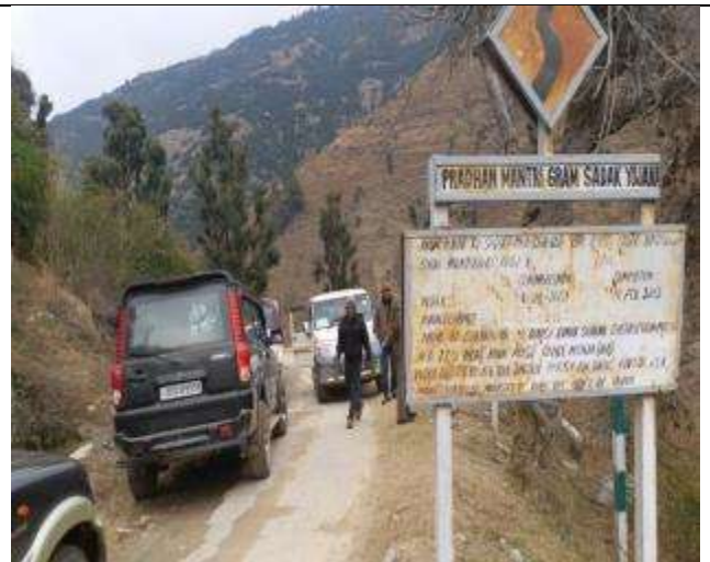
End Point, PMGSY Road Start at Ch 9.400 Km (Puneja Villa)
