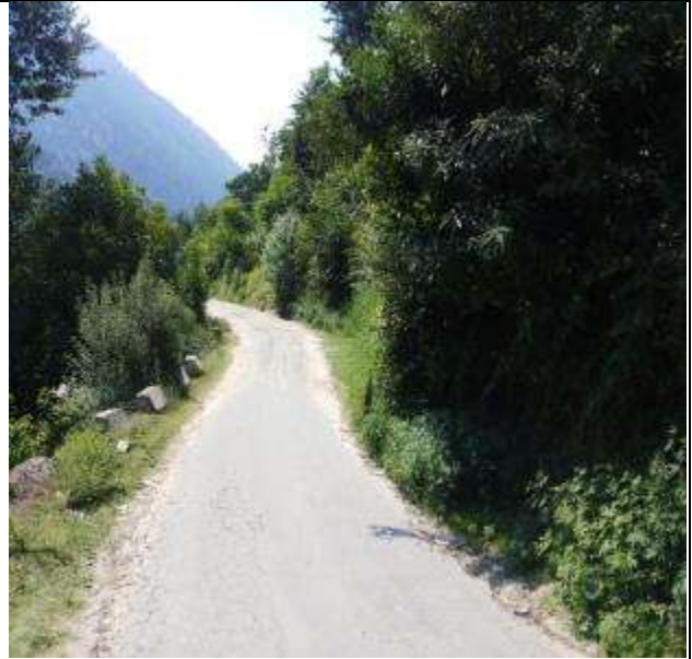
Condition of Existing Road
