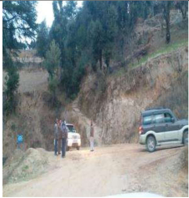
End Point Chainage-10.3 km
