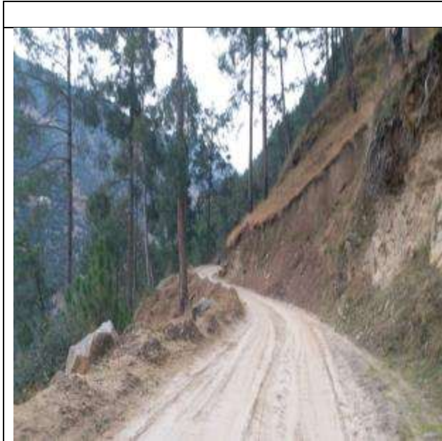
Condition of Road at Ch 5.1 km
