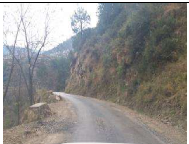
At Ch 1.500 Km
