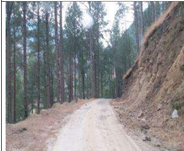
Trees close to the shoulder at Ch 7.000 Km
