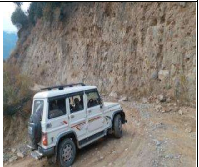
Sharp Turning and Poor Gradient at Ch 5.100 Km
