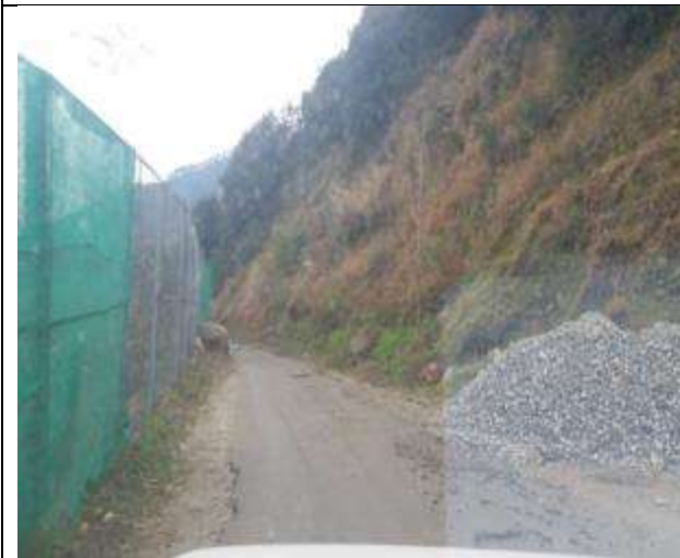
Army Camp from Ch 0.00-0.700 km
