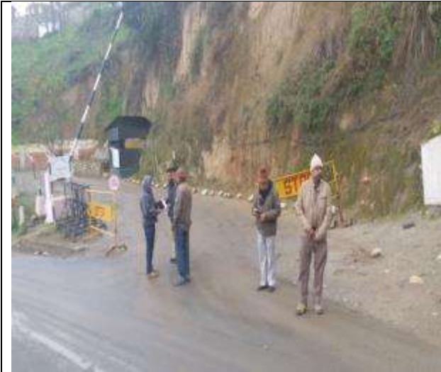
Condition of Road at Ch-0.00 km
