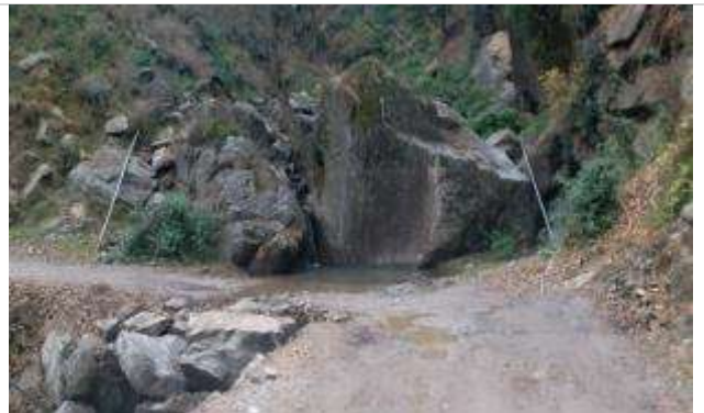
Erosion area Ch 8+100
