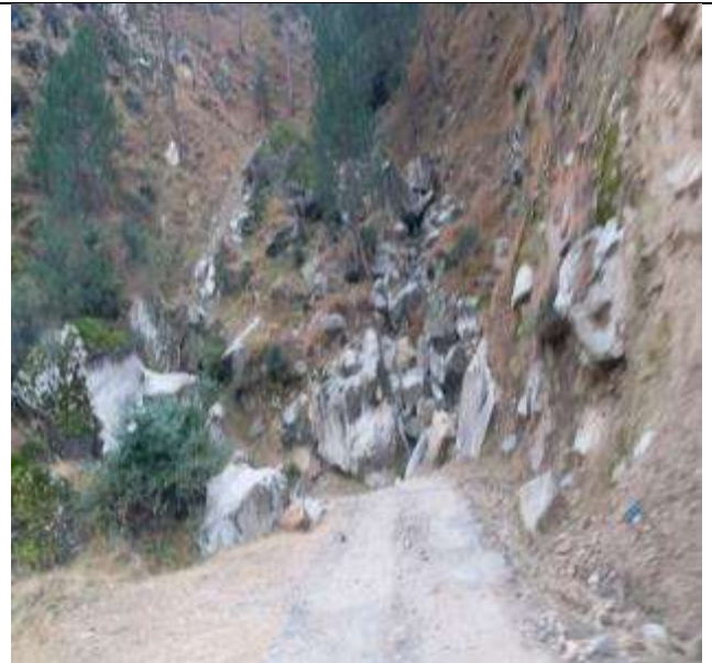
Land slide area at Ch 6.100 Km
