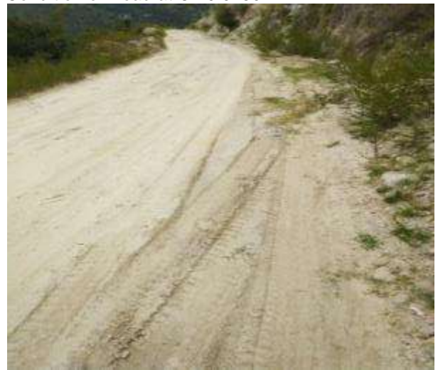
Condition of Road at Ch 0.200 Km
