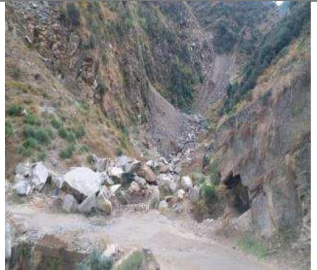
Causeway with Sliding Area at Ch 2.250 Km
