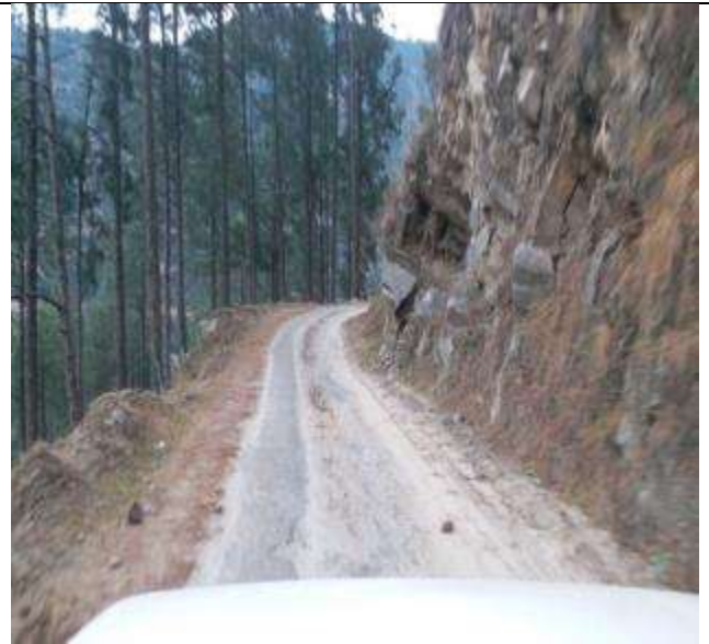
Photos show the trees close to the shoulder at Ch 5.400 Km
